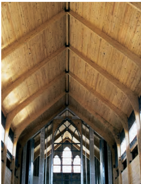
Church, Palm Beach Gardens, Fla., Unit Structures
