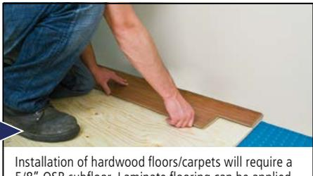
Installation of hardwood floors/carpets will require a 5/8" OSB subfloor. Laminate flooring can be applied directly on top of DMX 1-Step.
