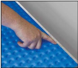
Keep a 1/4" gap between the sheet and wall to allow space for drywall or trim.
