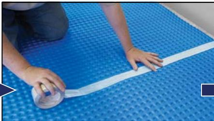
Tape seams together with sheathing tape, eliminating gap or overlap.
