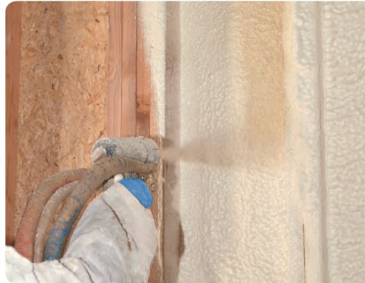
Spray Foam Insulation
