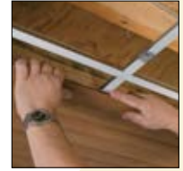
Position planks; slide and secure clips
