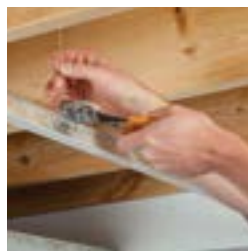
2 Suspend main beams with hanging hardware
