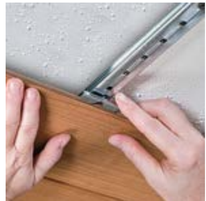
WoodHaven™ plank installation using Easy Up® tracks and clips
